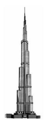
The construction of the Burj Khalifa required groundbreaking engineering and technological innovations. To support its immense height and withstand the harsh desert climate, the building incorporates a reinforced concrete core and a steel exoskeleton. The exterior is clad in reflective glass panels, which not only provide stunning panoramic views but also help regulate interior temperatures and reduce energy consumption.
